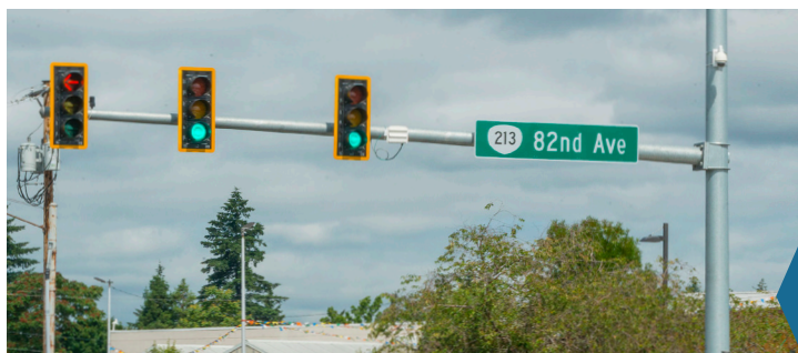
Safety improvements include upgrades to traffic signal heads with reflective backplates for improved visibility and safety.
